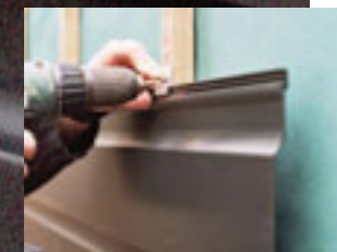
Planks fixed in full lengths, with staggered joints.
