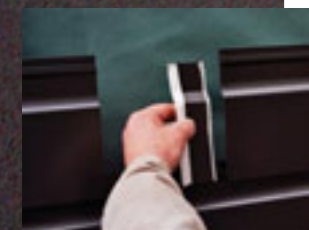
Insert joint plate with butyl tape
